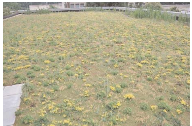
Photo 7 - Eight Months After Installation
