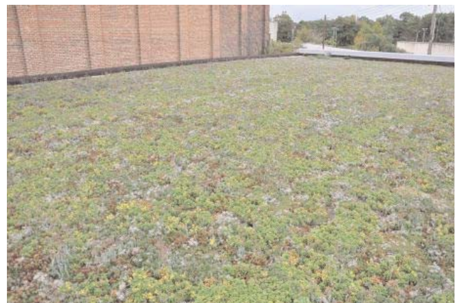
Photo 8 - One Year After Installation
