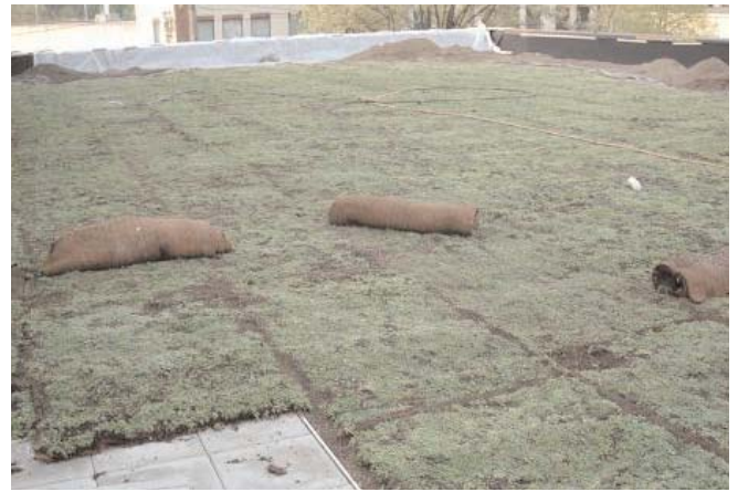
Photo 5 - First Day of Installation
