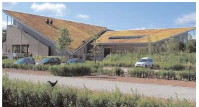
Photo 3 - Sloped Roof Application
