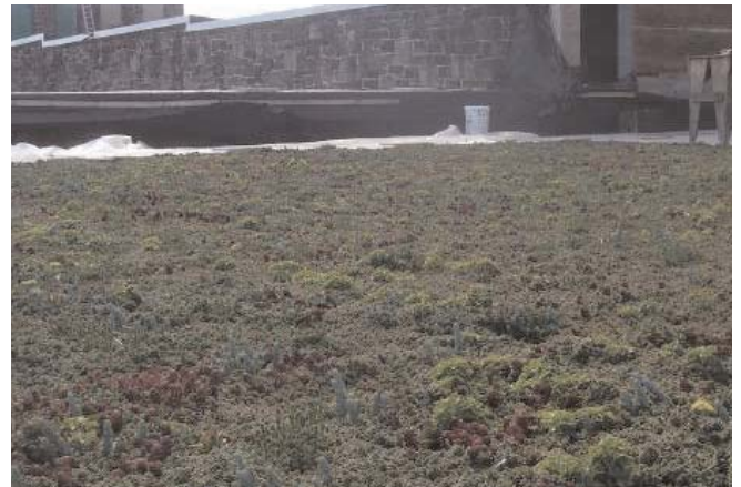
Photo 6 - Four Months After Installation
