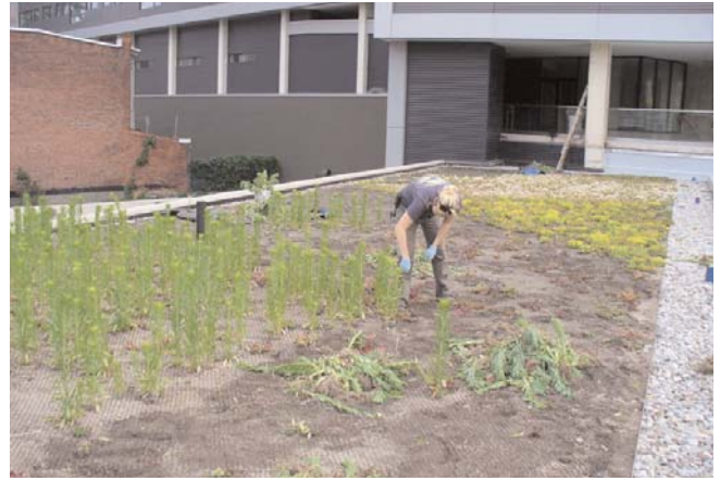
Photo 14 - Grown-on System 6 months following installation
