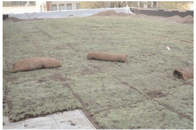
Photo 5 - First Day of Installation
