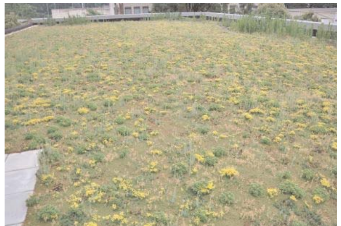
Photo 7 - Eight Months After Installation
