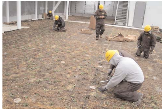
Photo 10 - Grown-on System during installation
