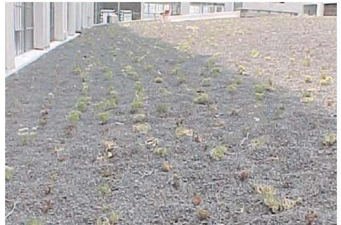
Photo 11 - Grown-on System after installation
