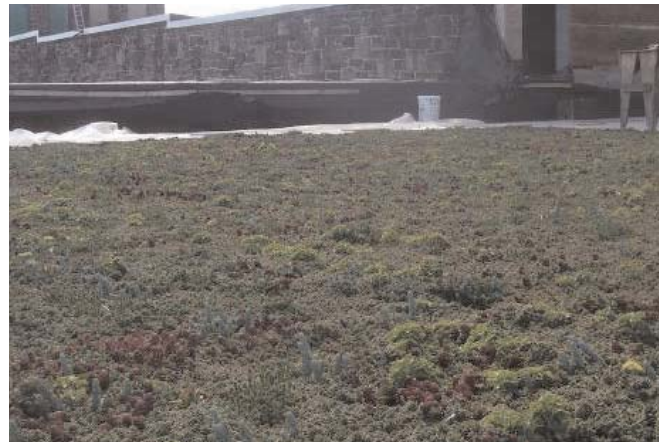
Photo 6 - Four Months After Installation
