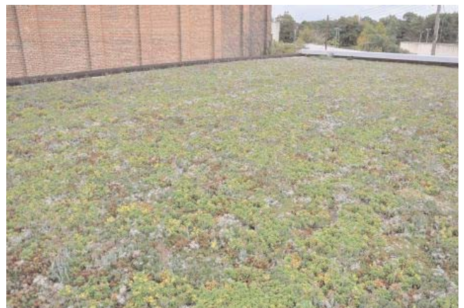
Photo 8 - One Year After Installation
